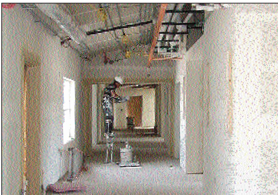
RIGHT: A worker on stilts prepares to do some mudding in the assisted-living area of the new facility. The area consists of 16 private rooms, each with a bathroom. It is being built to accommodate a 16-room addition in the future.
